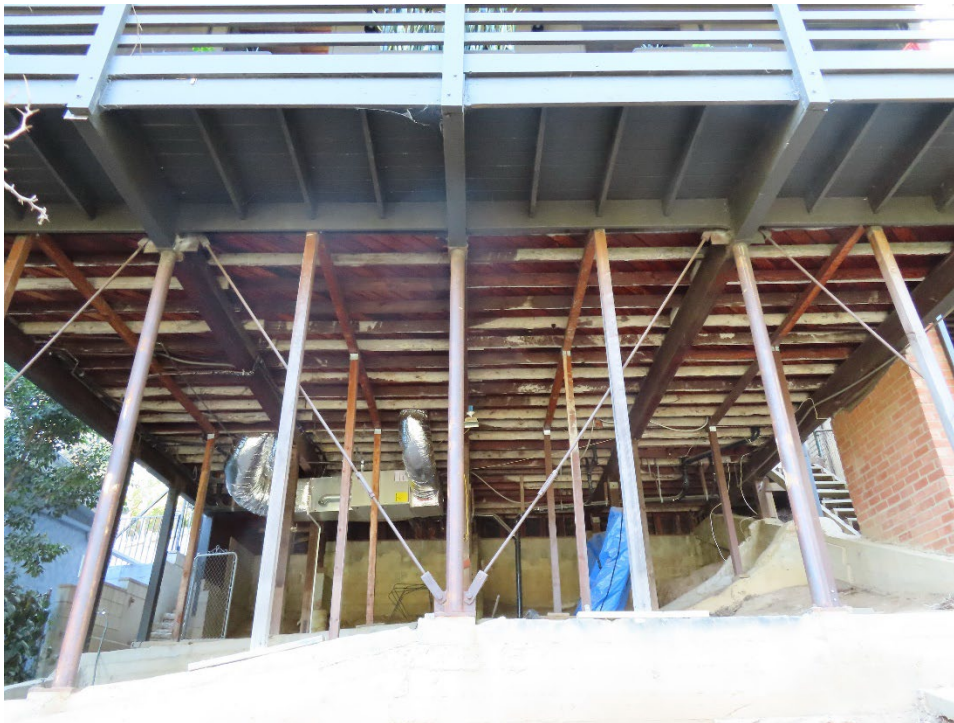
Photo 4 Foundation piers, view north (Architectural Resources Group)
